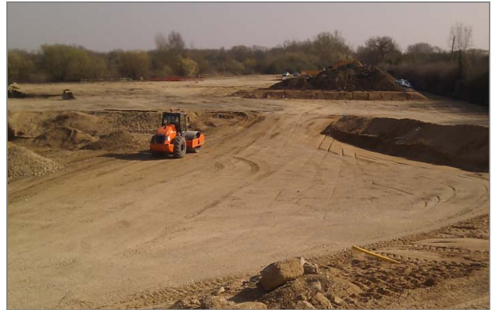
COMPACTION OF ENGINEERED FILL
