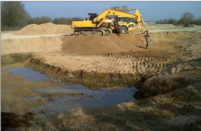
REMOVAL OF CLEAN OVERBURDEN
