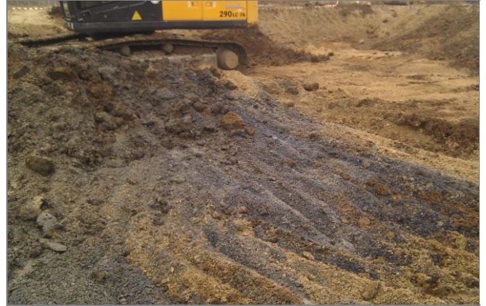
EXCAVATION OF HYDROCARBON IMPACTED GRAVELS
