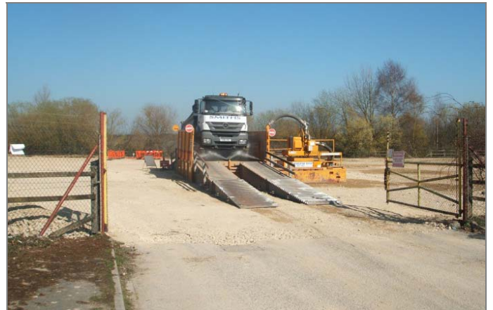
WHEEL WASH IN USE DURING REMOVAL OF MATERIALS
