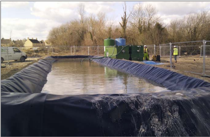
INSTALLATION AND TESTING OF WATER TREATMENT PLANT
