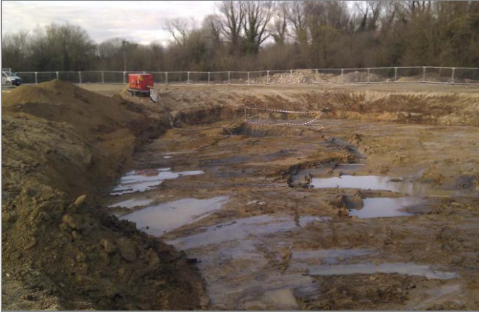
EXCAVATION FOLLOWING REMOVAL OF CONTAMINATION
