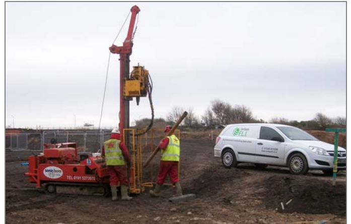
INSTALLATION OF SPARGE AND VAPOUR EXTRACTION WELLS
