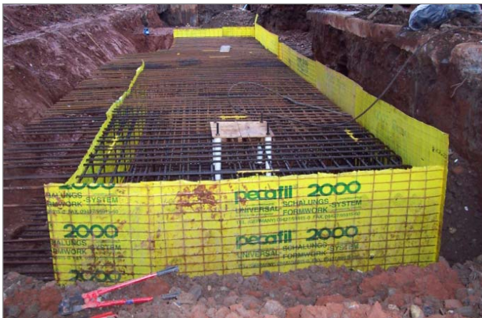
SHUTTERING TO PILE CAP
