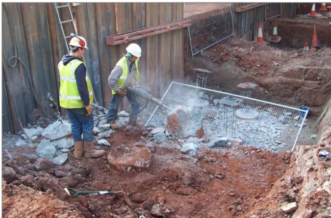
BREAKING PILE CAPS
