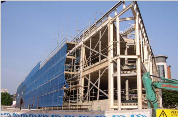
STEEL FRAME CONSTRUCTION
