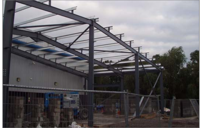
STEEL FRAME ERECTED
