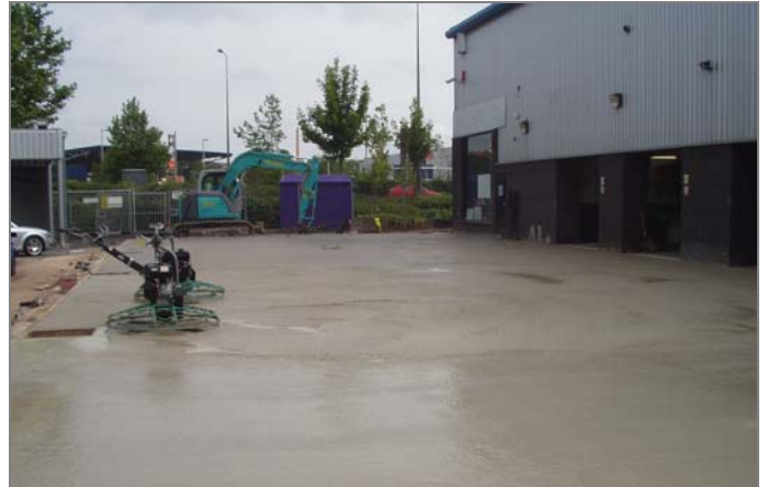
FINISHING CONCRETE
