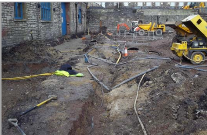
TRIAL PIT – MEASURING DEPTH
