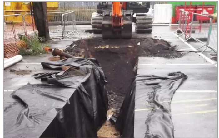
INSTALLATION OF STORM WATER DRAINAGE IN ACM
