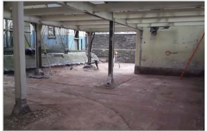
INDOOR EXCAVATION AREAS REINSTATED WITH CLEAN STONE
