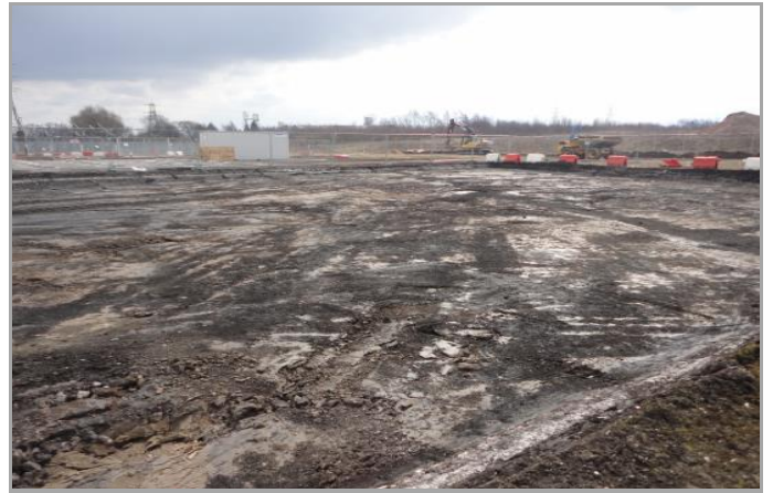
SECTION OF EXCAVATED CONTROL ZONE
