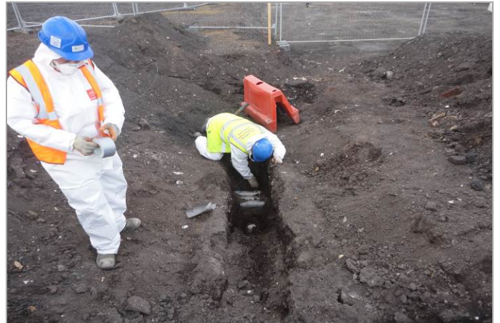
HAND EXCAVATION AROUND LIVE SERVICES
