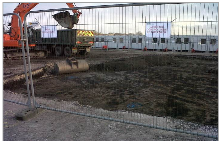
LOADING CONTAMINATED SOILS FOR OFF-SITE DISPOSAL
