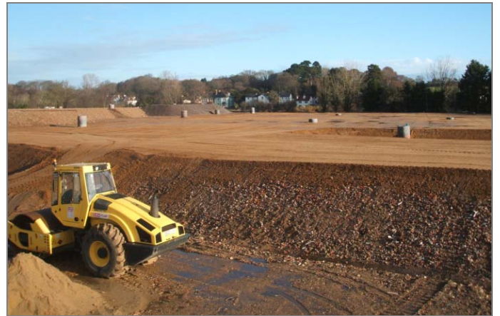
RAISING OF SITE LEVELS WITH ENGINEERED FILL
