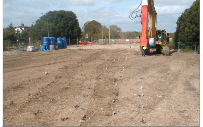
INSTALLATION OF BAND DRAINS
