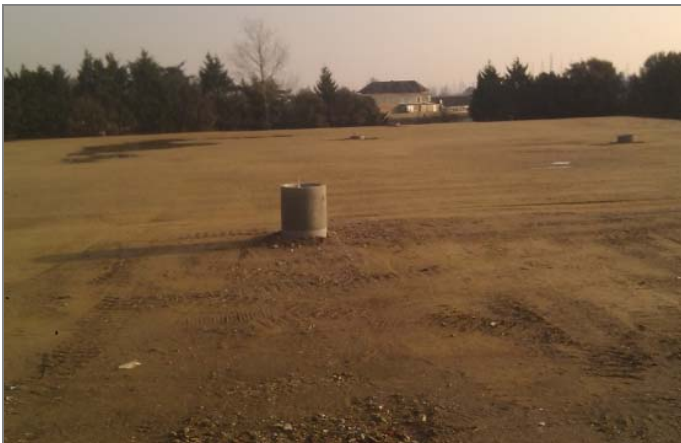
SETTLEMENT MONITORING POINTS BROUGHT UP IN CONCRETE RINGS WITH ENGINEERED FILL
