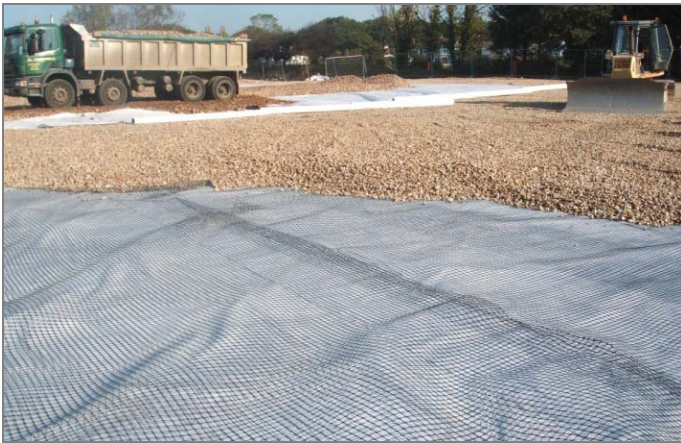
PLACEMENT OF ENGINEERED FILL ON GEOMEMBRANE AND GEOGRID
