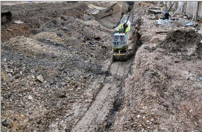
INSTALLATION OF PERIMETER CLAY STANK TO PREVENT EX-BOUNDARY RE-CONTAMINATION
